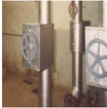
Figure 1 – Quick release valve insulation box for easy service access.
